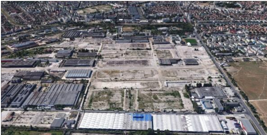
former "Tractorul Brasov" factory (> 130 hectares)
